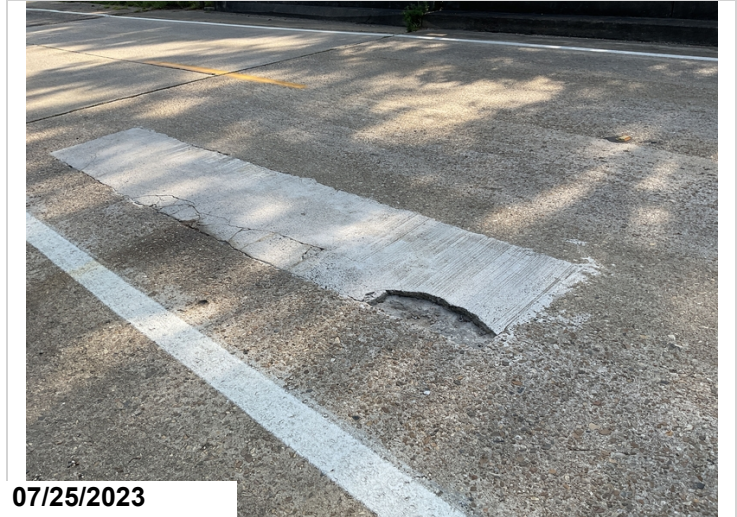
Deck span 3 left has spalling at previously patched area.
