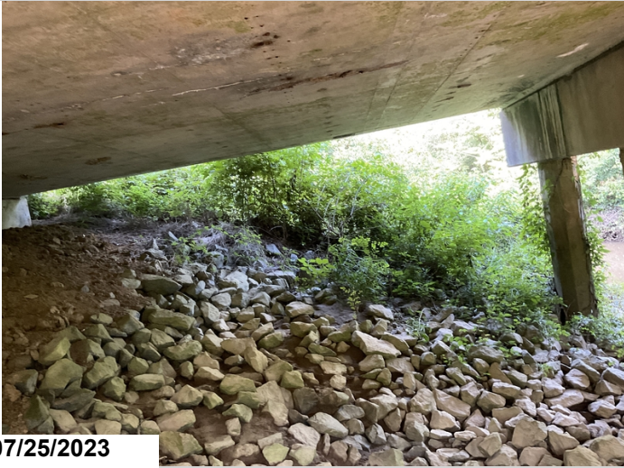
Span 1 left has trees, vines and vegetation impeding inspections.
