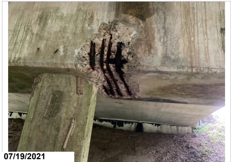
Bent 3 cap has spalls with exposed rebar. near pile 4.
