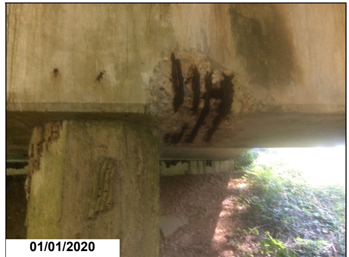
Bent 3 right of pile 4 spall with reposed rebar.
