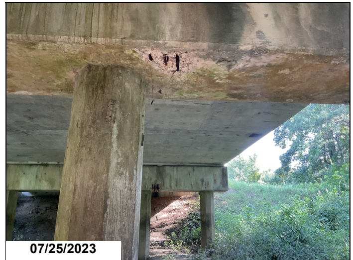
Bent 2 bottom of cap between piles 4 & 5 has spall with exposed rebar.
