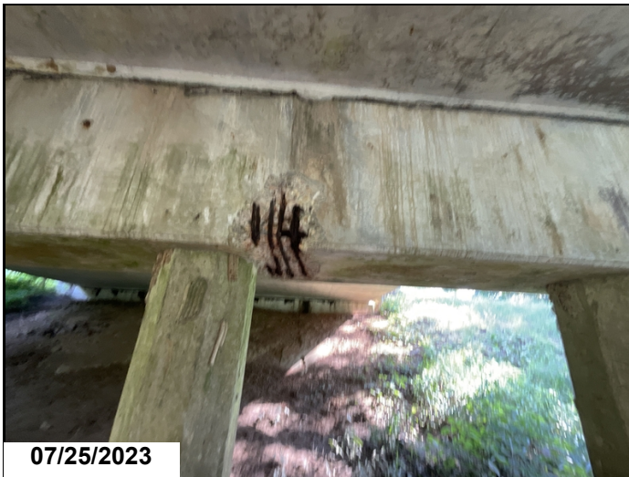
Bent 3 cap back between piles 4 & 5 has large spall with exposed rebar.
