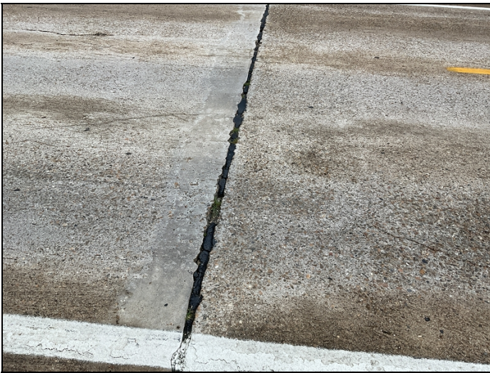
Bent 2 joint material has missing areas with loss of adhesion and debris impaction.
